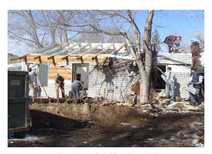
*Image 6. Deconstruction of home in Lyons, Colorado following buyout.* This deconstruction project took place following major flooding along the Saint Vrain River in Lyons, Colorado. *Image: Gavin Smith.*
